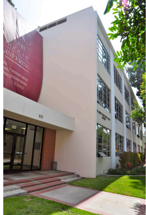
Neely Petroleum and Chemical Engineering Building
